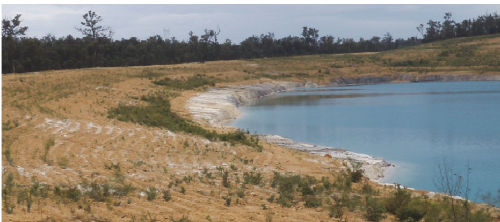
Figure 1 An extensively 'rehabilitated' 20 year old pit lake in southwest Western Australia showing the limited catchment of some pit lakes (bounded by the tree line) and the difficulty in predicting final rebound heights. Final water height is at least 2 m below that predicted, reducing the value of much of the bankside contouring for development of a littoral and riparian margin
