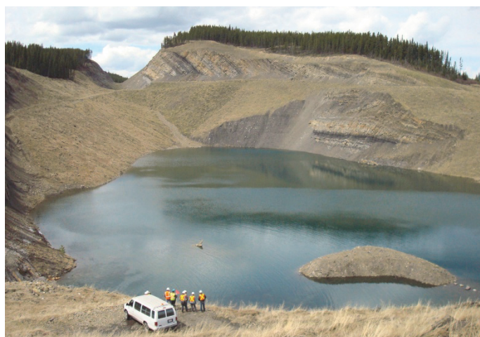
Figure 5 Sphinx Lake, Alberta – A pit lake designed and implemented by Teck Coal that includes littoral habitat that is 23% of total surface area and other habitat enhancements; the lake supports rainbow trout ( Oncorhynchus mykiss ) and bull trout ( Salvelinus confluentus )
